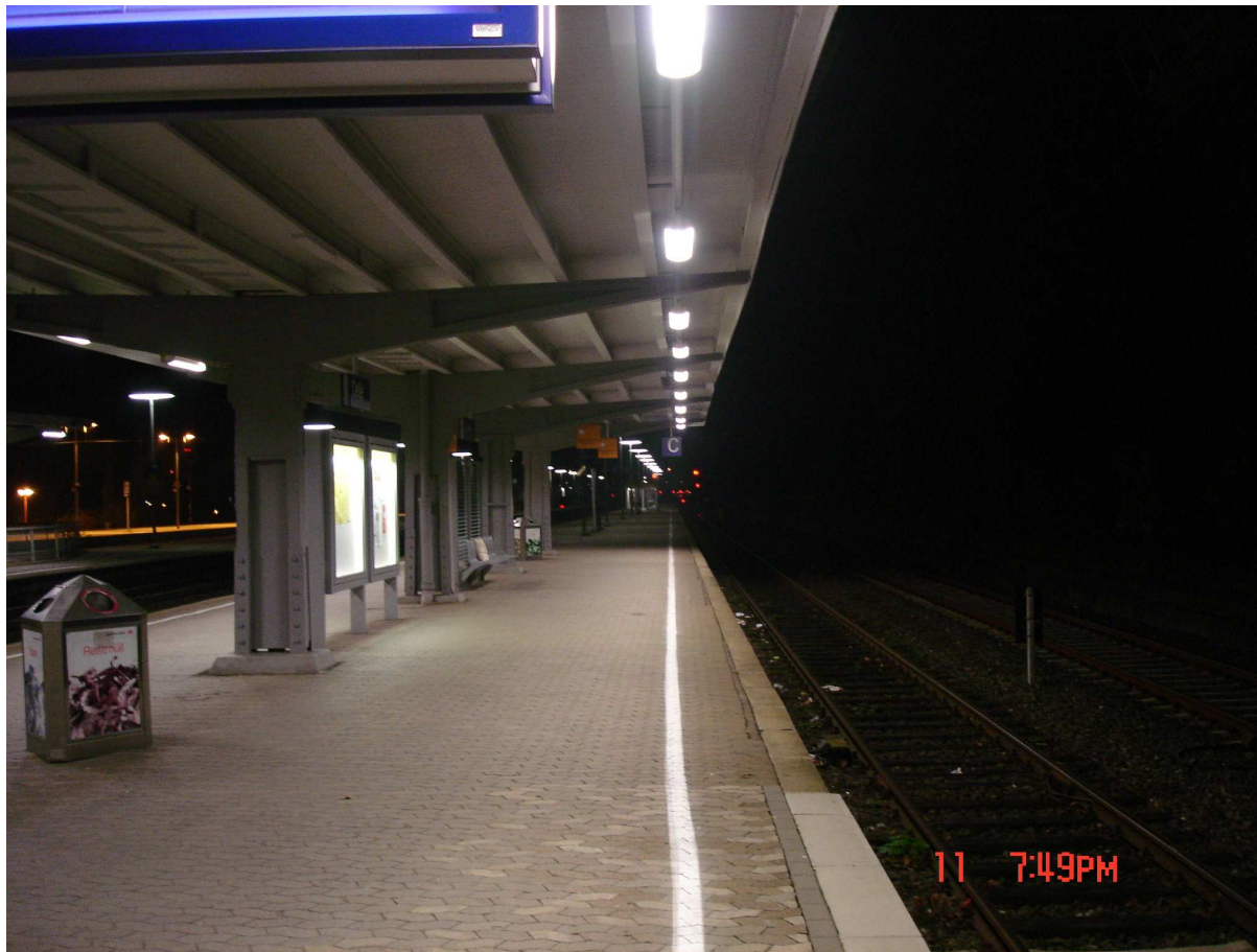
Celle, fluorescent night time lighting
