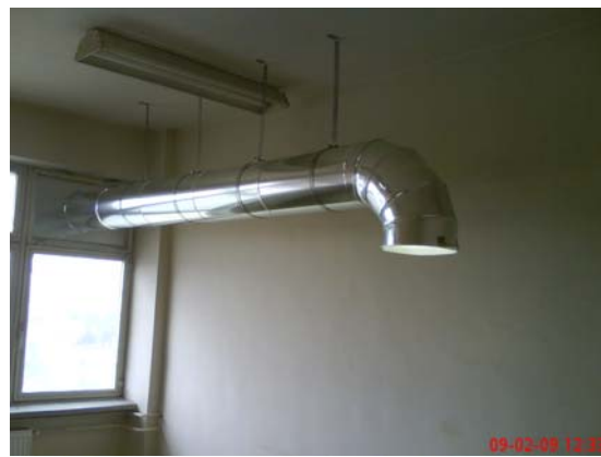
Figure 4 Horizontal SunPipe ending with two 45 degrees elbows above imaginary false ceiling.
