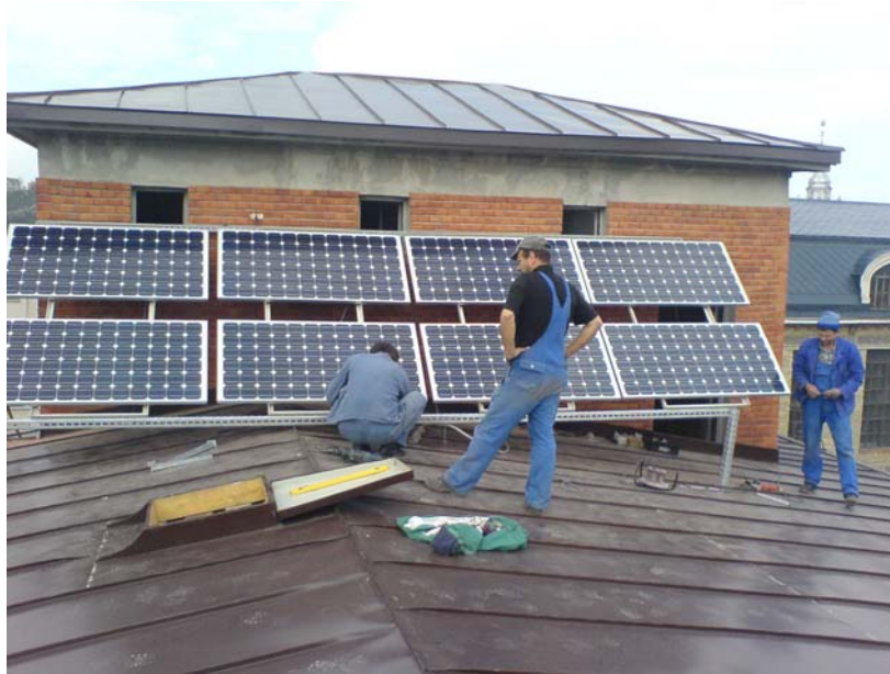
Figure 8 Mounting the panels
